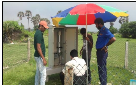
Fig.4.3. Remote monitoring stations at Thalai Mannar
